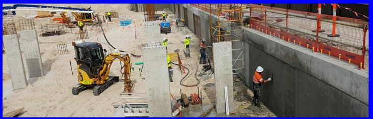
A smooth Class 2 steel trowel surface finish offers a cost effective alternative design by eliminating the additional step of cladding / rendering wall surfaces.
