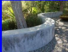
Sprayed concrete has no restrictions on shape or size, so free-form shapes such as curved walls and unusual designs are no problem at all.
